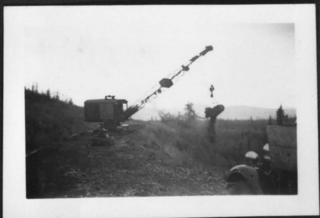
90 ton, 1/2 yard, dragline cleaning out the ditch.
