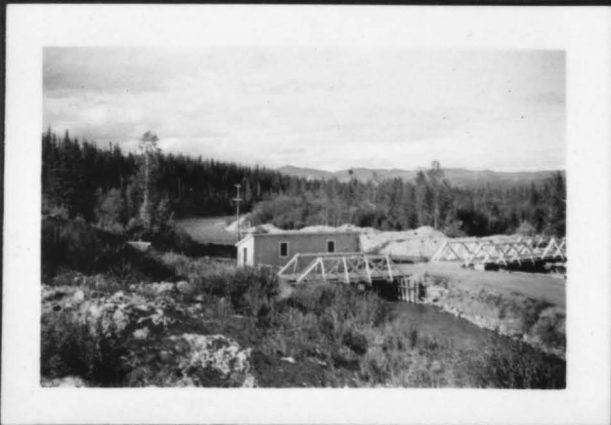
North Fork Intake
