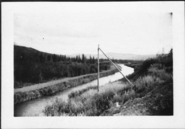
North Fork Power Project Ditch.
