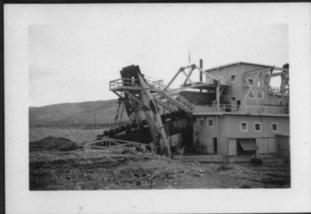
#8, Middle Sulphur, stops a few minutes for repairs.
