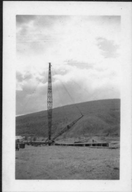
Another "bow frame" goes in place.
