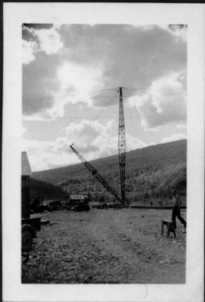
115' mast, 100' boom 25 ton cap., derrick.
