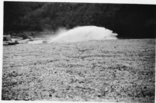
A "Giant" (monitor) eats a path thru the tailings for the new #4 dredge.
