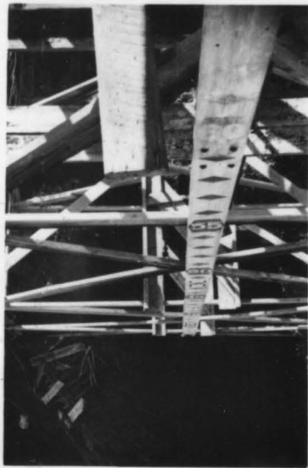
Depth gauge to a $800,000 earth fill reservoir for Bunker Hill workings.
